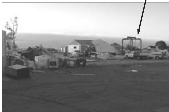
Little remained of the Northern Plains warehouse after the tornado hit around 10 p.m. Fortunately, the facility’s containment system held the 3,200 gallons of Round-up that leaked from a broken seal on a stainless steel tank.
