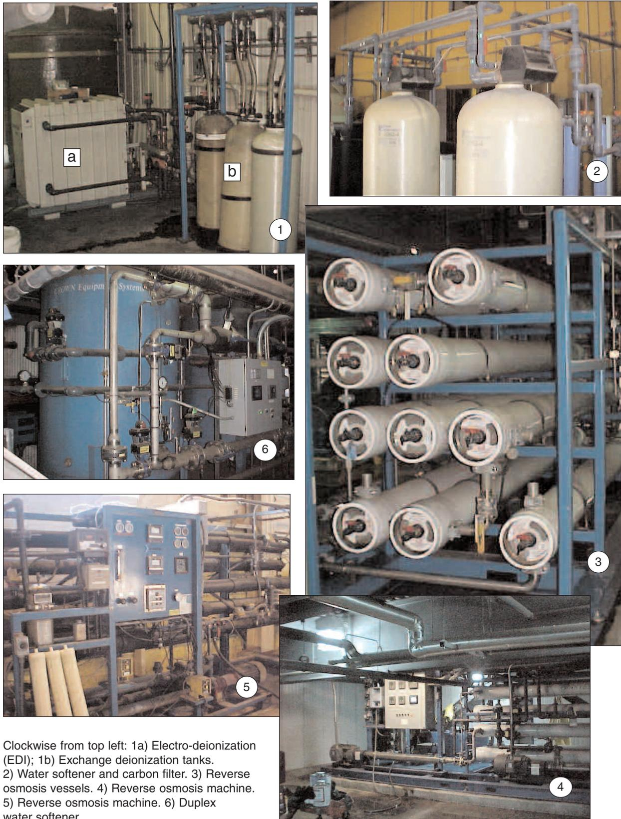
Clockwise from top left: 1a) Electro-deionization (EDI); 1b) Exchange deionization tanks. 2) Water softener and carbon filter. 3) Reverse osmosis vessels. 4) Reverse osmosis machine. 5) Reverse osmosis machine. 6) Duplex water softener.
